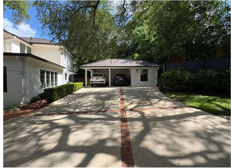
514 Patterson South Elevation of Existing Carport & Guest House (Main House shown to Left)
