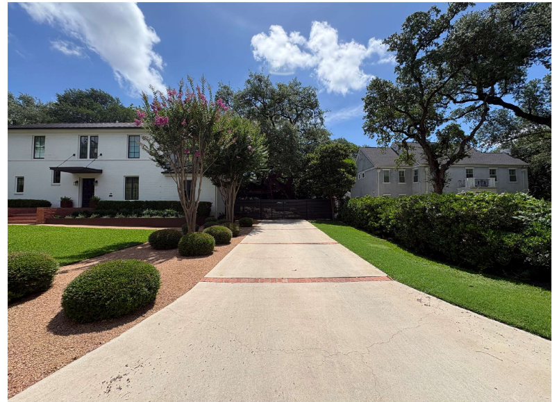
514 Patterson Front Elevation from Driveway
