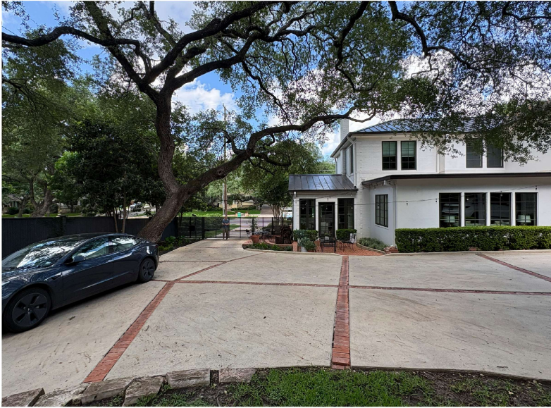
514 Patterson East Facade Viewed from Rear Yard
