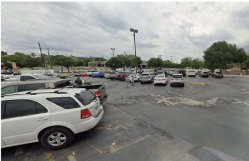
Existing Parking Deck
