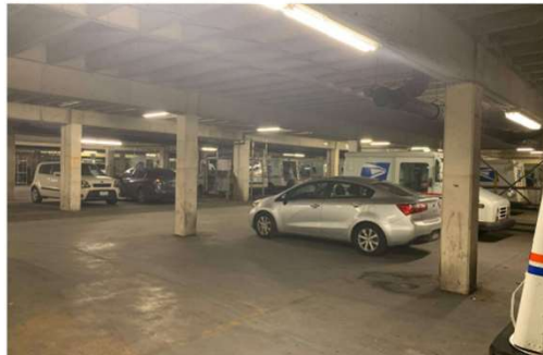
Existing Underground Parking
