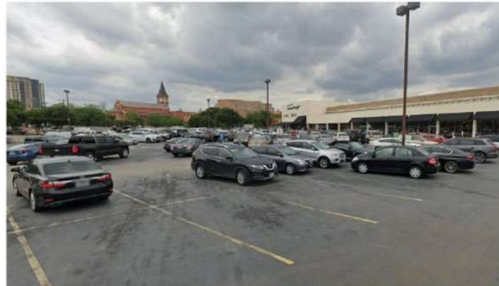
Existing Parking Deck
