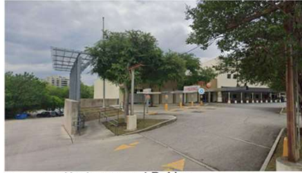
Ramp To Underground Paking
