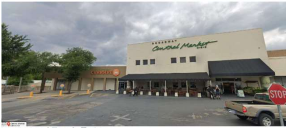
Curbside / Fresh Entry
