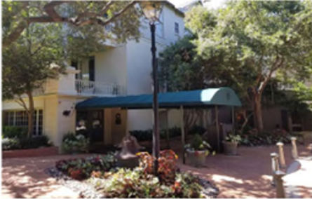
Existing Building Side View
