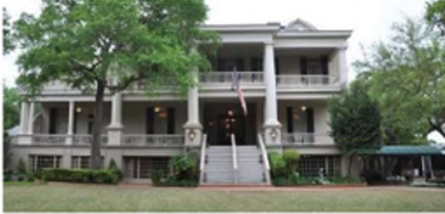
Existing Building Front Entry
