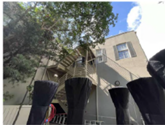
Existing Building Back Stair
