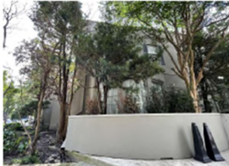
Existing Building Back View
