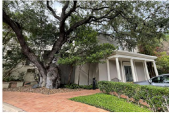
Existing Building Side View
