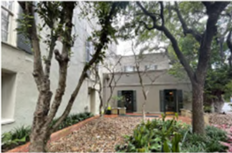
Existing Building Side View
