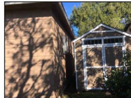
EXISTING STRUCTURE - EAST
