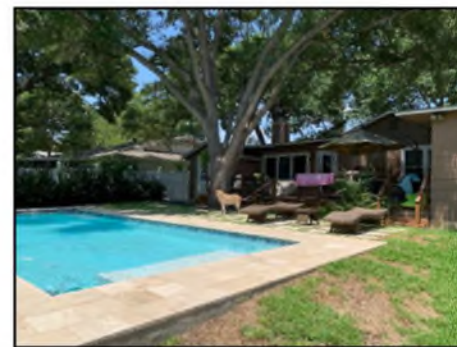
EXISTING STRUCTURE - SOUTH
