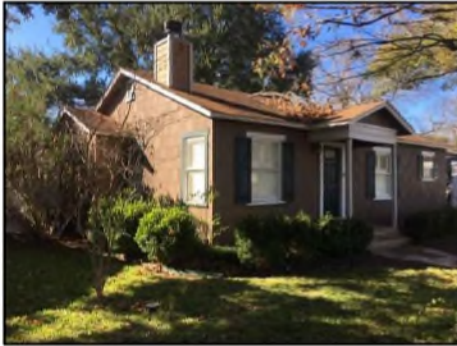
EXISTING STRUCTURE - NORTH
