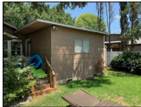
EXISTING STRUCTURE - SOUTH
