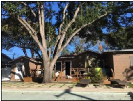
EXISTING STRUCTURE - SOUTH
