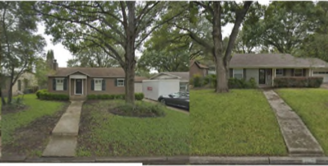
PROJECT SITE EXISTING SINGLE-FAMILY RESIDENCE TO BE DEMOLISHED. EXISTING FRONT-FACING GARAGE NOT SETBACK PER ZONING.
