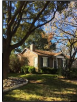
EXISTING STRUCTURE - NORTHEAST
