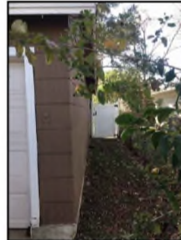
EXISTING STRUCTURE - WEST
