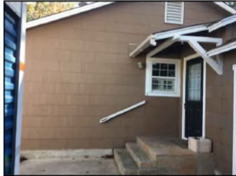
EXISTING STRUCTURE - WEST
