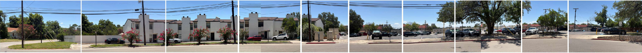
GROVE PLACE FACING SOUTH
