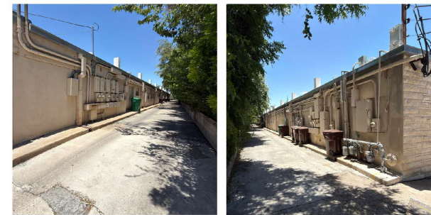
ACCESS DRIVE FACING WEST
