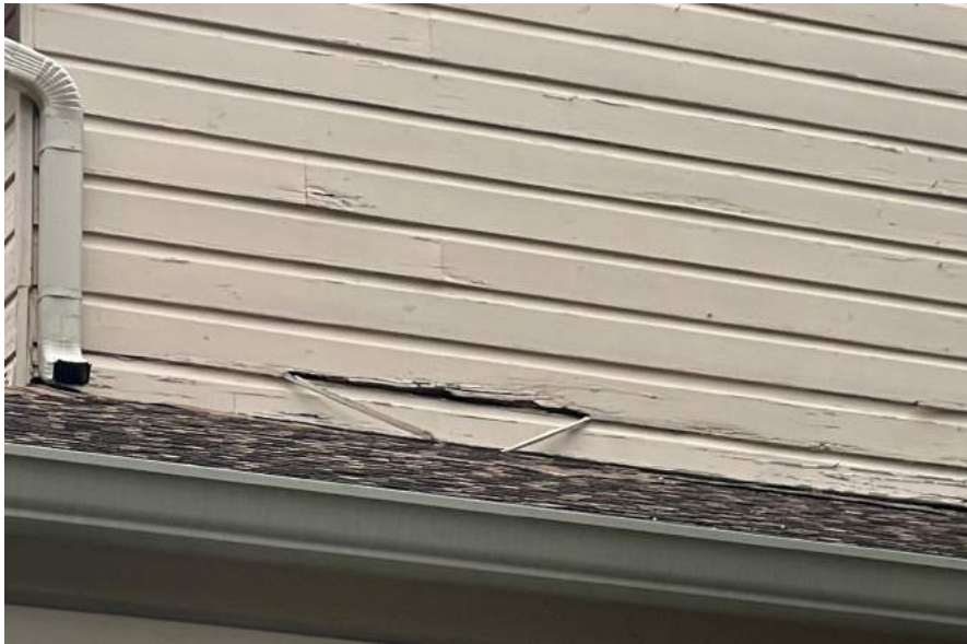
MOISTURE INFILTRATION DAMAGE to SIDING - TYPICAL
