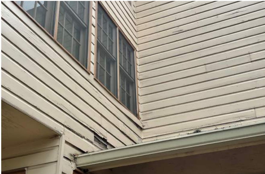
WOOD-ROT and DECAY - TYPICAL ALL ELEVATIONS
