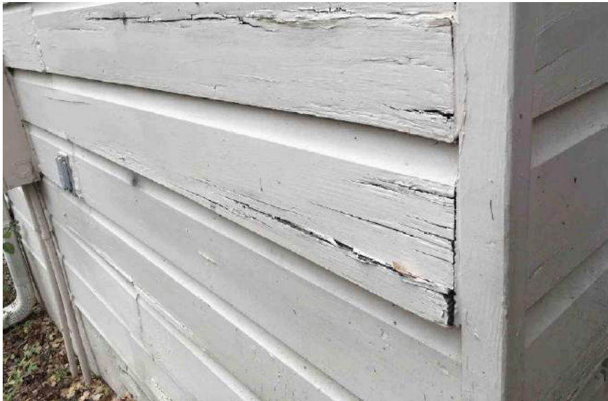
EXTENSIVE WOOD-ROT and DECAY - TYPICAL
