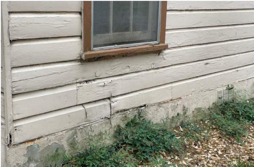
MOISTURE INFILTRATION - PROMOTES MOLD GROWTH
