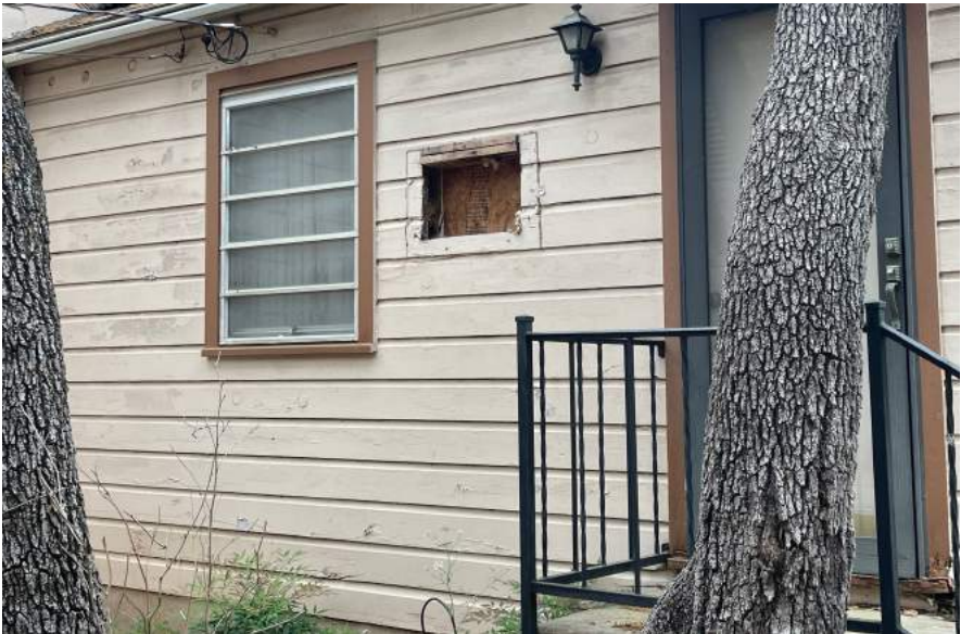
EXPOSED WIRING and EXT. WALL CAVITY
