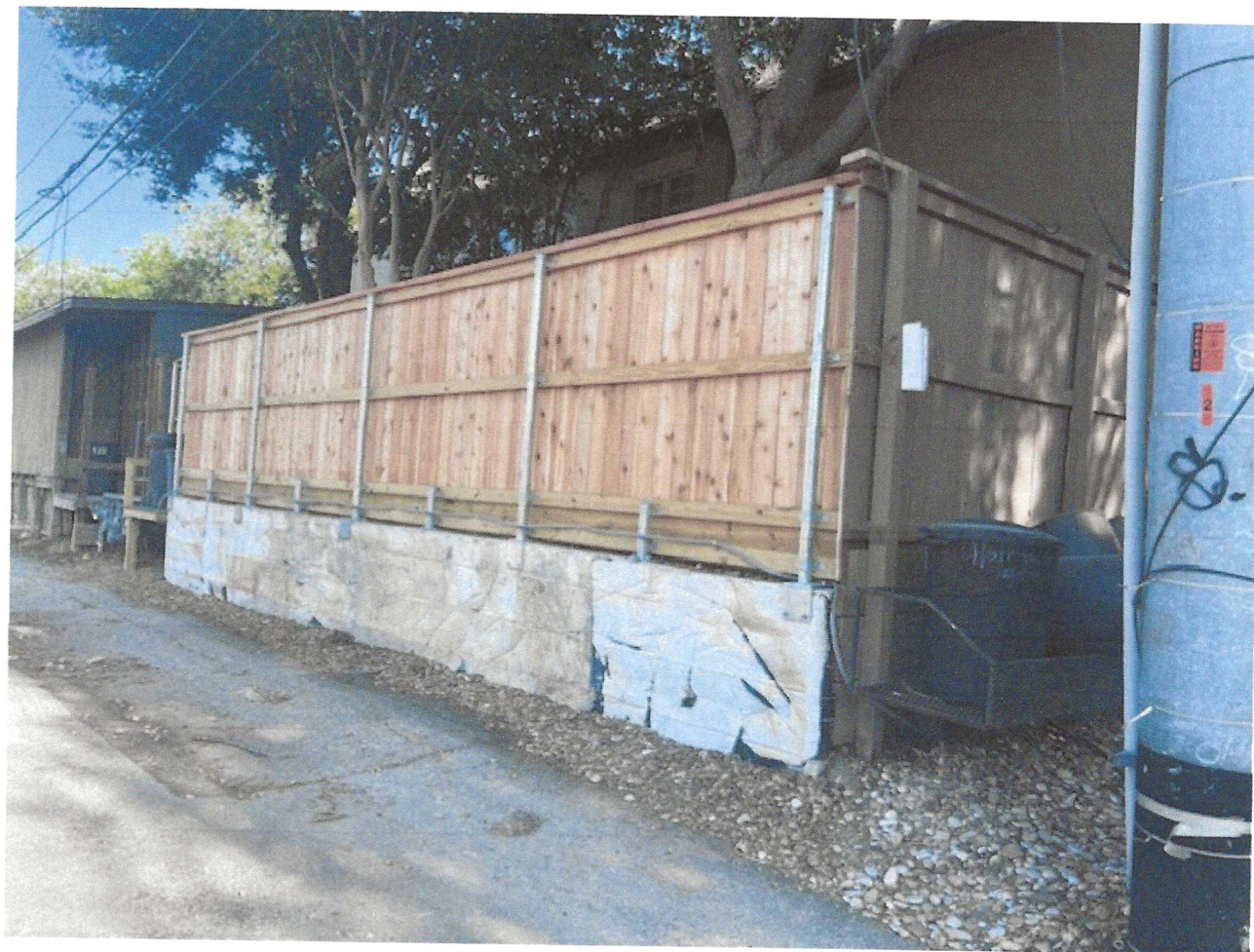
The new 6 foot fence was constructed on top of the concrete retaining wall and meets the side fences that have not been replaced.
