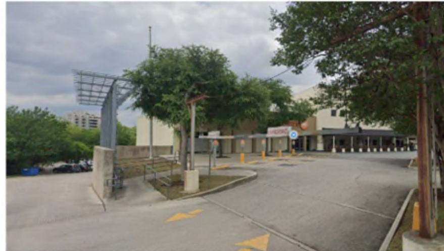
Ramp To Underground Paking
