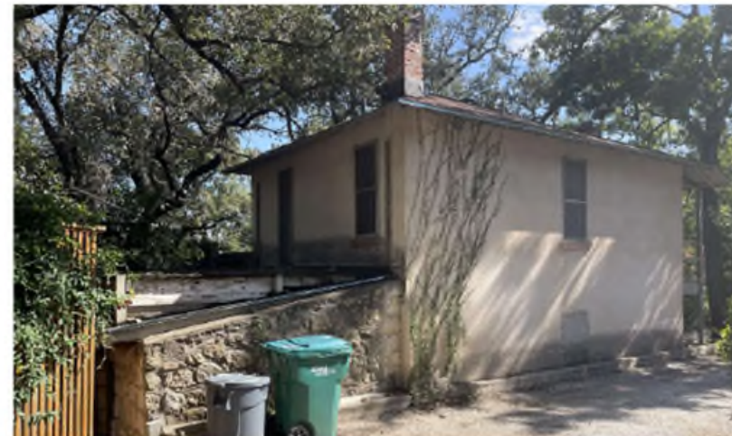
NORTHWEST ELEVATION DETACHED STRUCTURE
