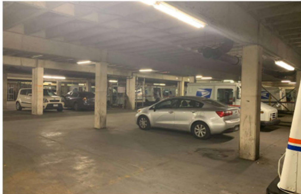
Existing Underground Parking
