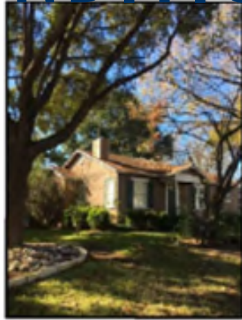
EXISTING STRUCTURE - NORTHEAST
