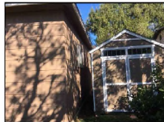
EXISTING STRUCTURE - EAST
