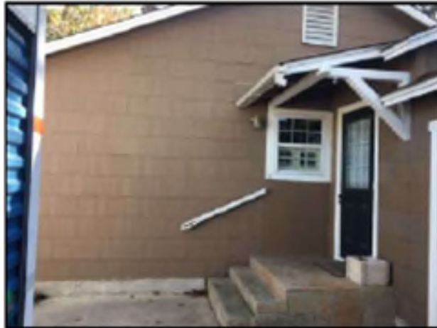
EXISTING STRUCTURE - WEST
