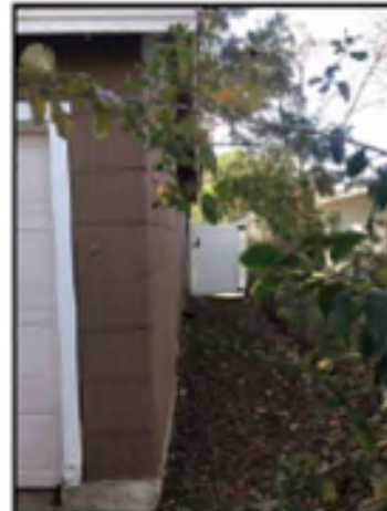
EXISTING STRUCTURE - WEST
