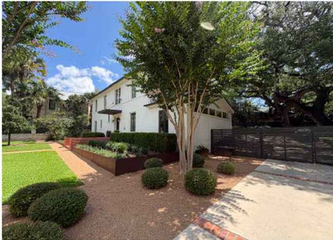
514 Patterson Southwest Corner of House at Driveway
