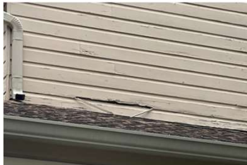
MOISTURE INFILTRATION DAMAGE to SIDING - TYPICAL
