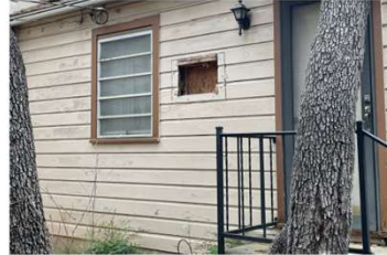
EXPOSED WIRING and EXT. WALL CAVITY
