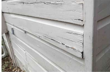
EXTENSIVE WOOD-ROT and DECAY - TYPICAL
