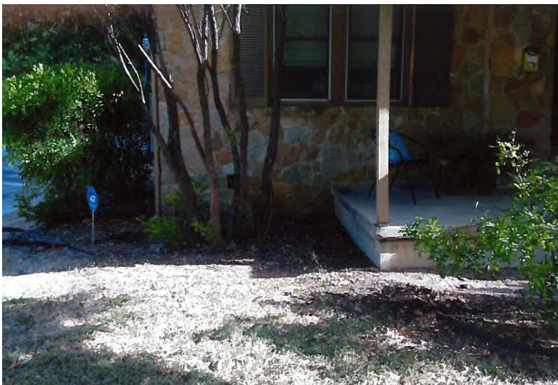
CLOSE VIEW OF FRONT PORCH
