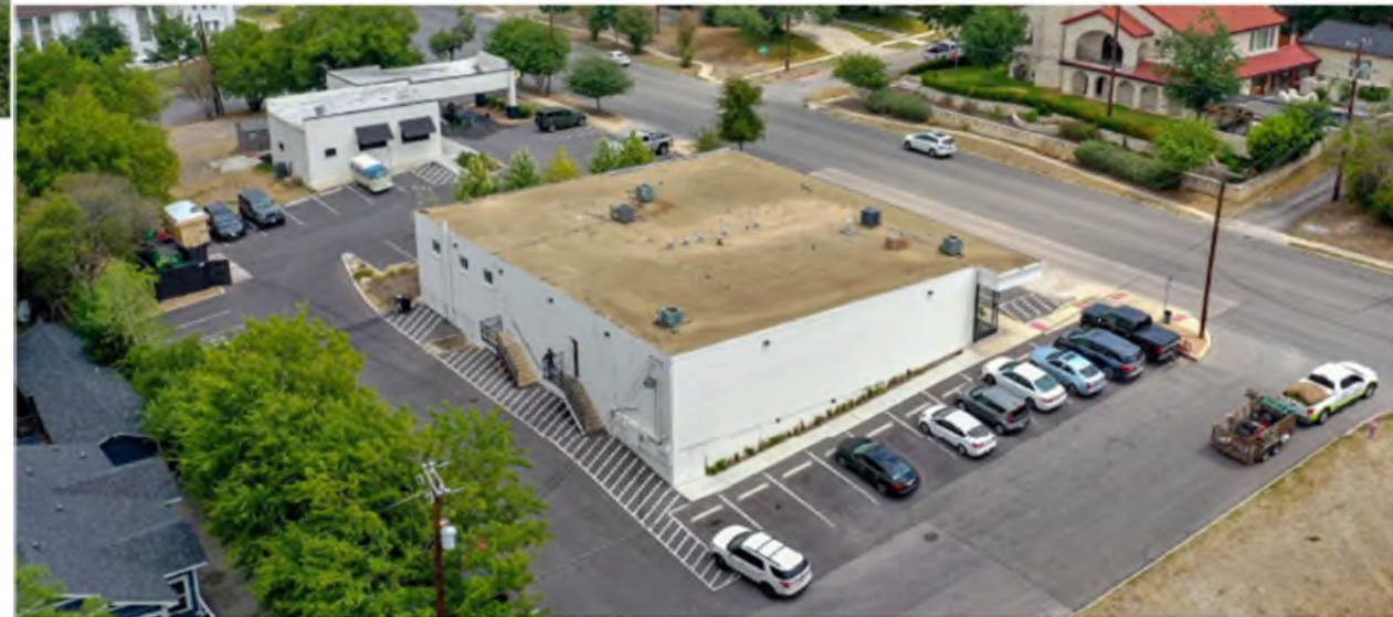
DRONE PHOTOGRAPHY FROM INSLEE VIEWING NORTHEAST
