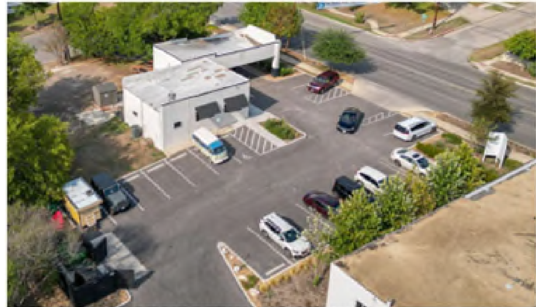
DRONE PHOTOGRAPHY OF AREA OF WORK VIEWING NORTHEAST
