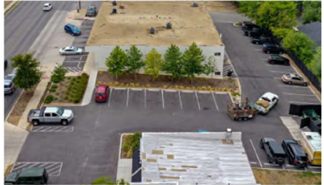
DRONE PHOTOGRAPHY OF AREA OF WORK VIEWING SOUTH
