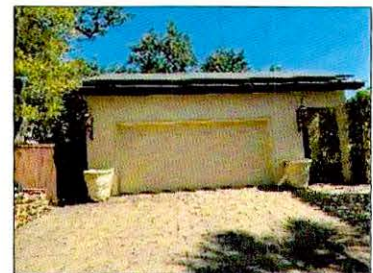
EXISTING GARAGE PICTURE 8-7-2023
