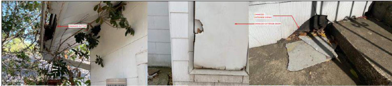
DAMAGED and RUSTED GUTTER
