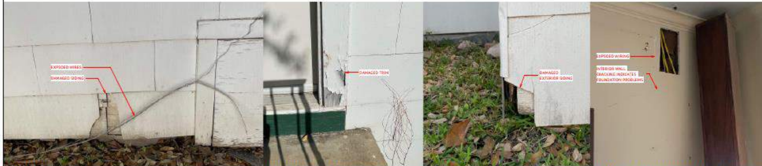
DAMAGED EXTERIOR SIDING
