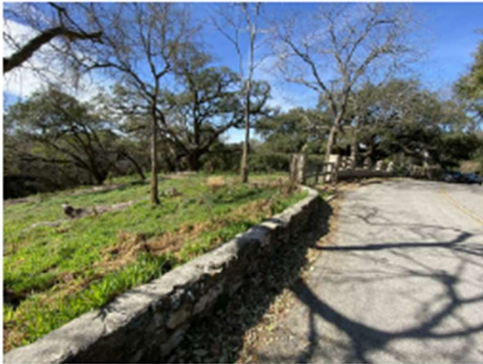
EXISTING 1920'S 2'-0" STONE WALL TO REMAIN
