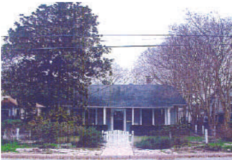
316 Argo before planned demolition
